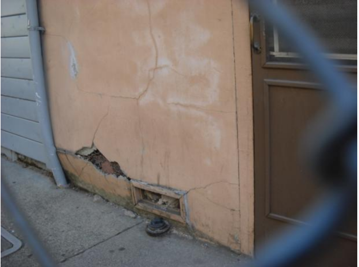
Photo 17: This is a photo of the Hangtown Tree Bar as seen from Center Street near Placerville City Hall. This structure was constructed of unreinforced masonry and has become significantly dilapidated to the point at which it requires a chainlink fence barrier. Several studies have been conducted on this building and most recently, it was identified as a threat to the health and safety of citizens beyond the proximity protected by chainlink fencing.
