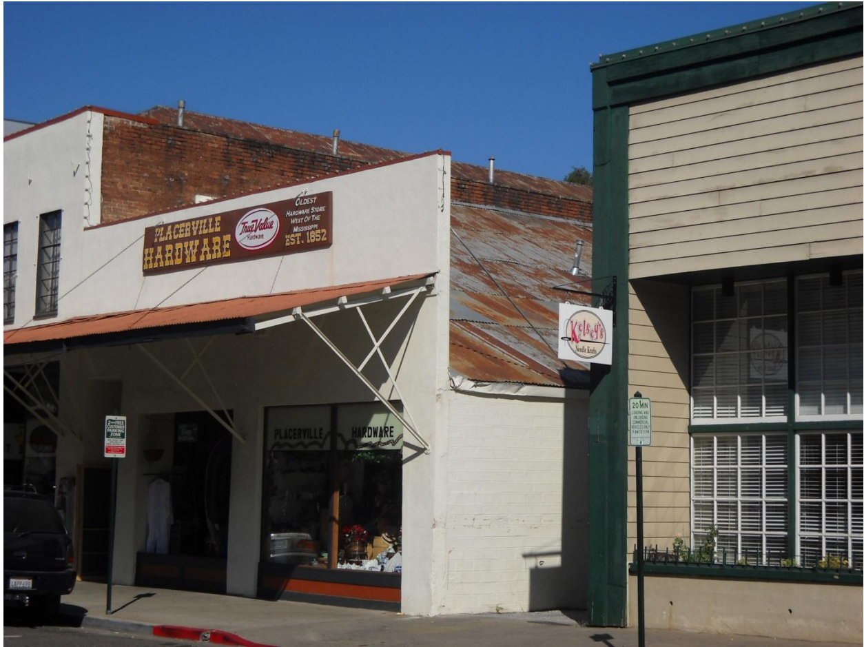
Photo 1: This is a photograph of 438 Main Street in Downtown Placerville, built in 1876. This unreinforced masonry building has damaged and deteriorated building materials due to lack of adequate weather protection. The corrugated metal roof is deteriorated and rusted. The bricks on the side exterior wall are damaged and portions have fallen away from the building.
