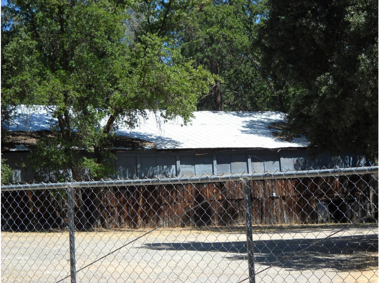
Photo 13: This structure was built in 1934 and was formerly used as a roller skating rink until it was boarded and deemed to be unusable by the City. It has dilapidated roofing, deteriorated eaves, and damaged exterior building materials. The structure has been fenced off and boarded to prevent persons from entering as it is unsafe to occupy.
