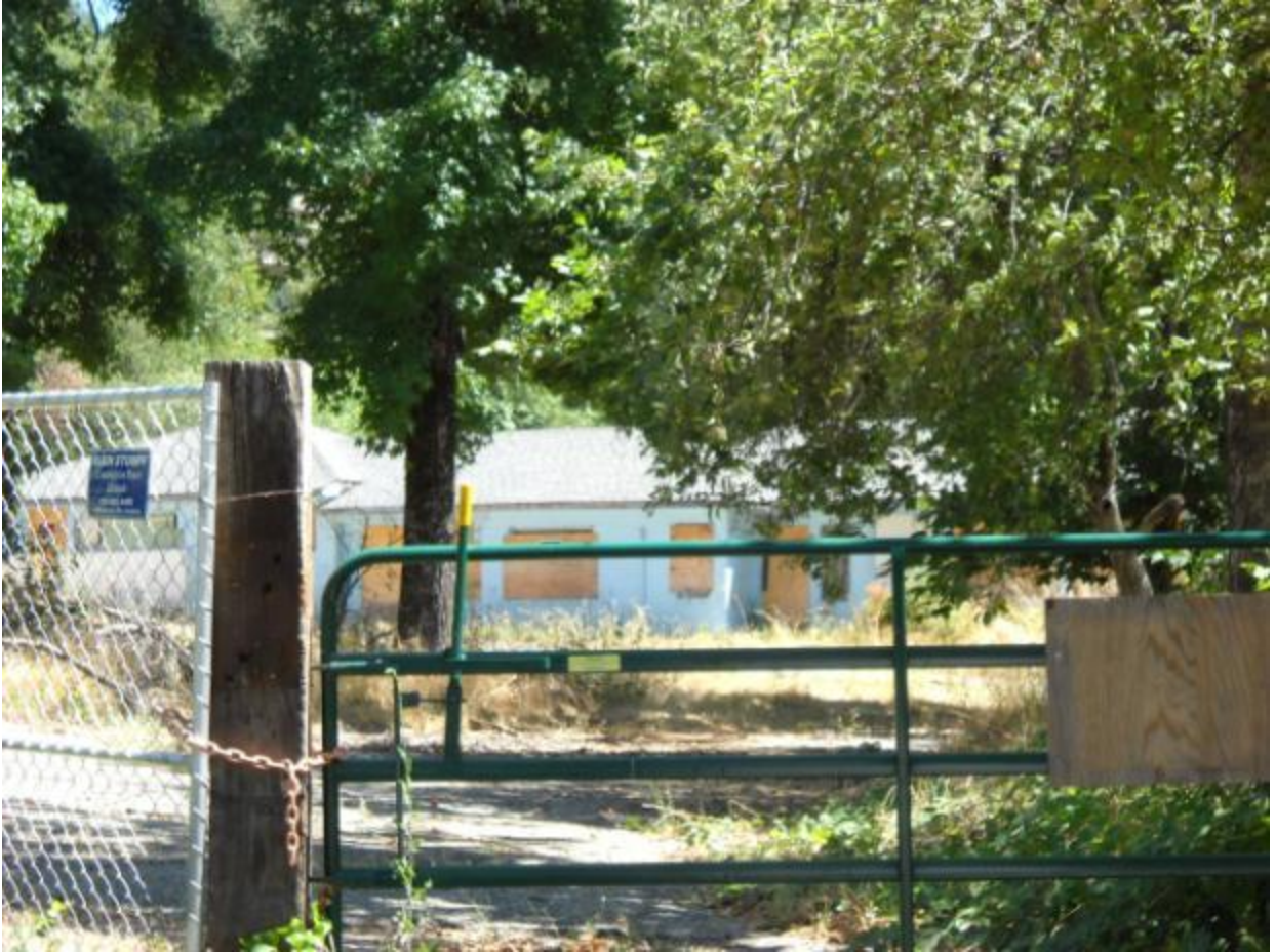
Photo 11: This is a vacant multi-family residential property located at 2100 Ferndale Court and built in 1952. The property has been deemed uninhabitable by the City due to major code violations. According to City staff, this structure was illegally converted from a single family dwelling to a multi-family residential property without permits or entitlements. Unpermitted construction represents a threat to the health and safety of occupants due to a lack of construction standards. The property was overcrowded and had excessive trash and inoperable vehicles on-site. There are several other boarded units behind the building shown in the photograph.
