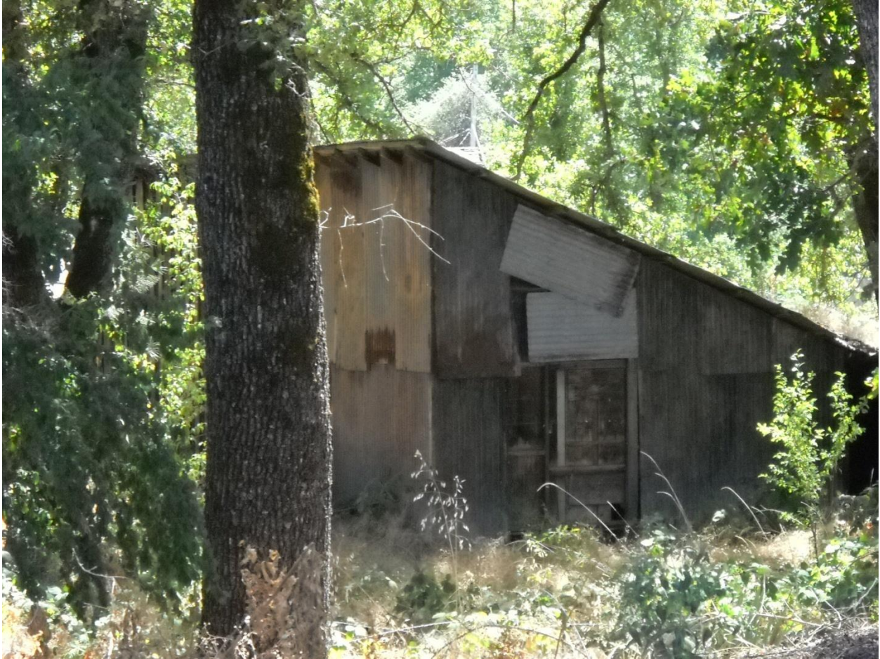
Photo 18: This structure is located on Alexander Court in the Smith Flat portion of the Project Area. Faulty weather protection has caused the exterior building materials, eaves, and overhangs to become damaged. The corrugated metal siding is warped and rusted and provides inadequate protection to interior building materials. Additionally, this structure does not have an in-tact foundation, which increases risk of collapse. These conditions make the structure unsafe to occupy.
