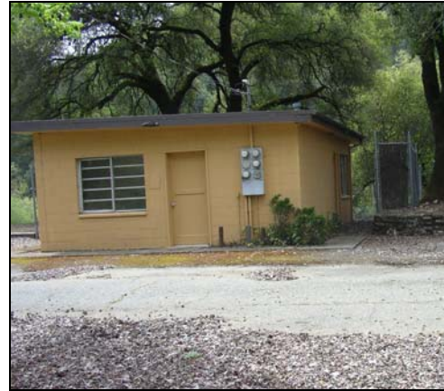
Existing restroom facility.
