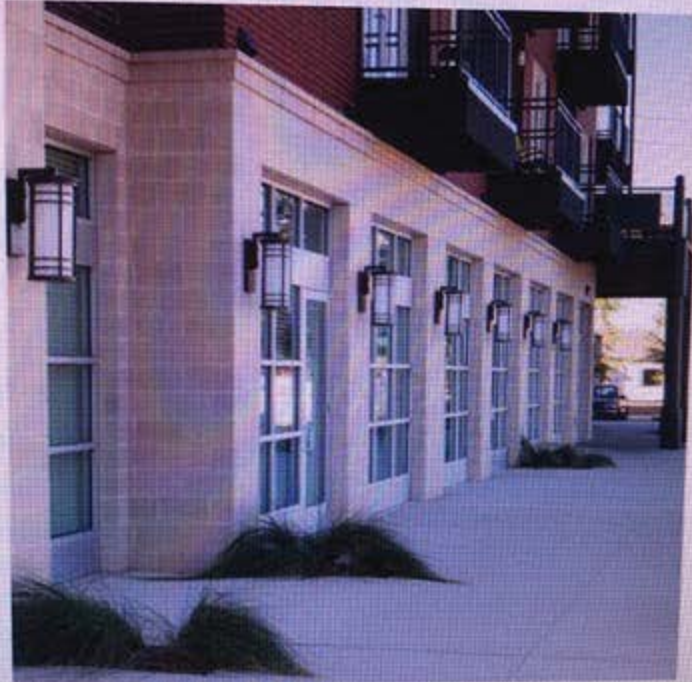
Solid materials, tall ceilings, frequent pilasters, divided glazing systems, special light fixtures, and a covered facade articulate spaces that can be either retail or residential. (JHP)
