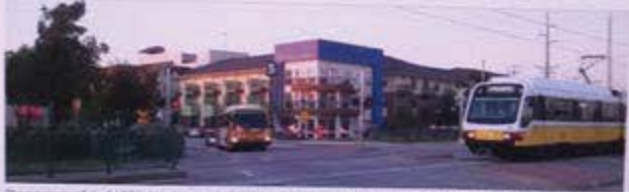
The proximity of the DART light-rail line, their frequent bus service, and the presence of retail shops along Fifth Street, with mixed housing above, help create a more urban environment for Doka 5th Street Crossing in Garland, Texas. (Jonathan Brown)
