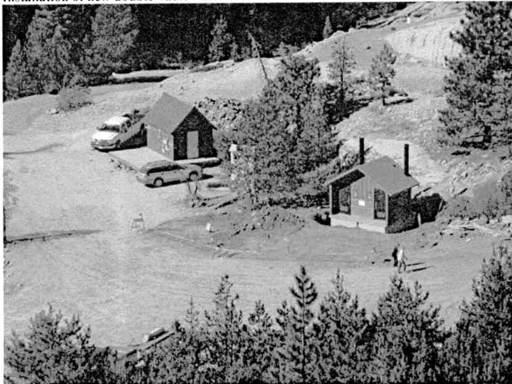
New restroom at Rubicon Trail Loon Lake Trailhead, installed in Sep. 2008 (foreground). Structure in background used to store outreach materials (e.g. trail brochures/maps, oil spill kits, cardboard commodes, “wag bags”) and for volunteers to handout to users.
