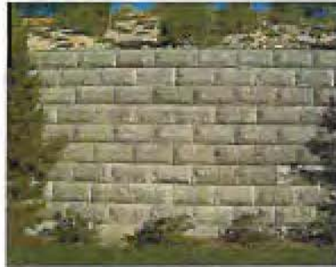
RETAINING WALL NO SCALE
