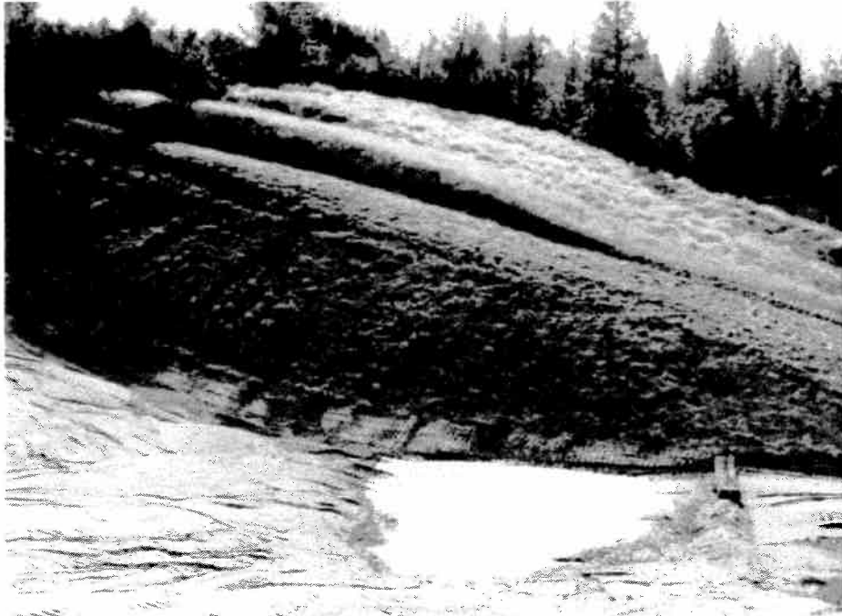
Photograph No. 5. View of imported and graded soil stockpile and sediment retention area. Toe of recent extraction area visible at lower left (viewing south).
