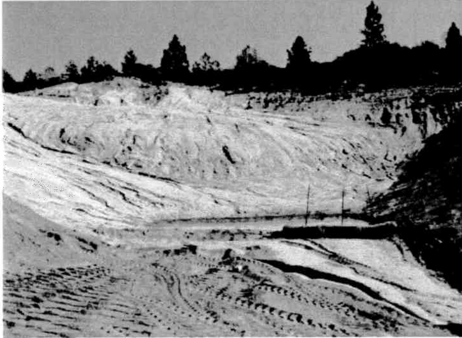
Photograph No. 7. Central pit showing working face of recent extraction area and sediment retention structures at center (viewing east).
