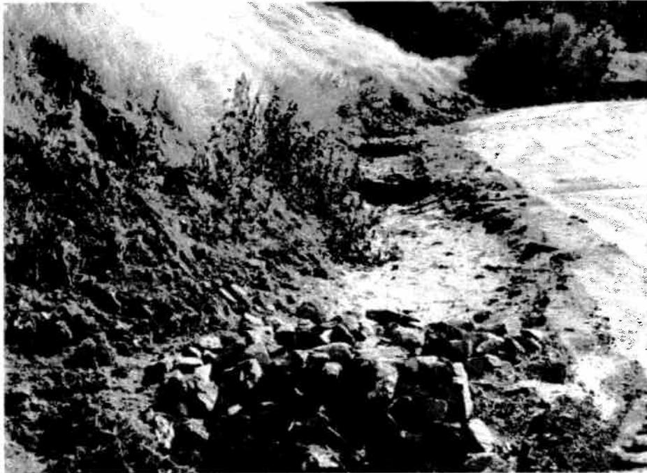
Photograph No. 11. Sediment check dams in drainage ditch at base of topsoil stockpile in western portion of quarry (viewing west).
