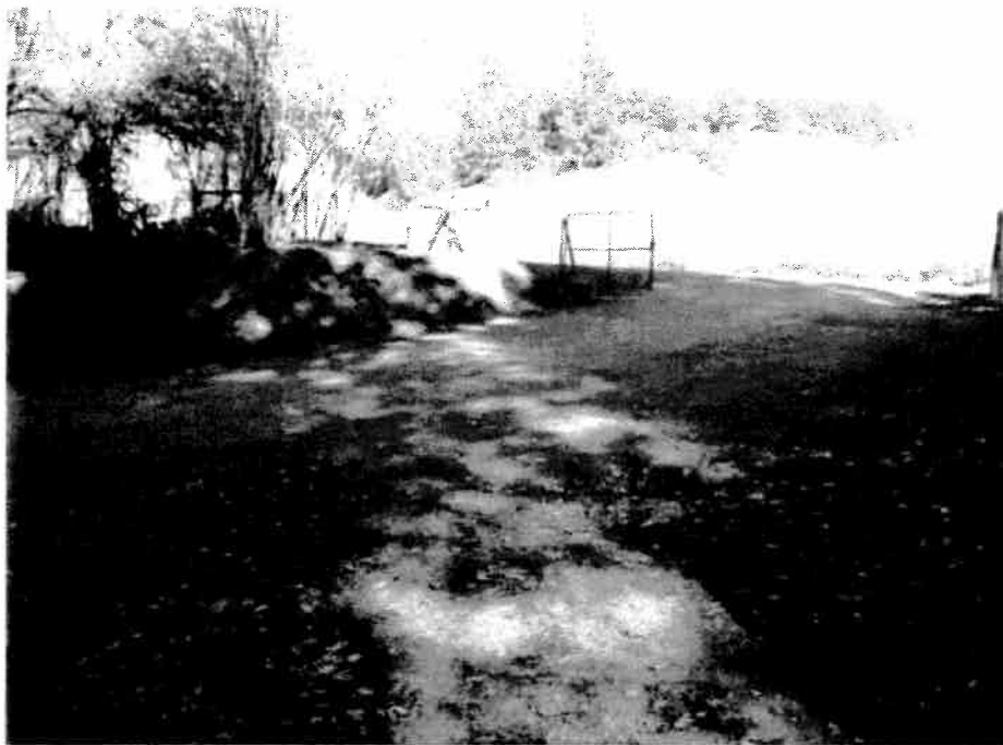
Photograph No. 2. Site entrance and equipment staging area adjacent to maintenance building along western site boundary. Portion of imported soil stockpile visible at upper right (viewing northeast).
