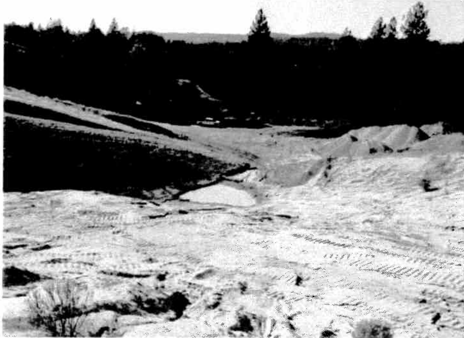
Photograph No. 3. Overview of quarry floor with sediment settling area in center, straw- and mulch-covered imported soil on left, material stockpiles at right, equipment maintenance and staging areas at center, and recent extraction area in foreground (viewing west-southwest).
