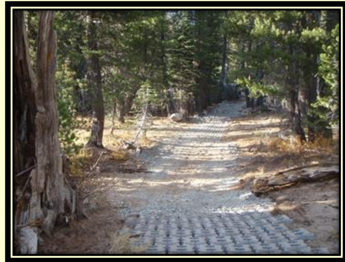
Completed block approaches to drainage crossings at Meadow 6 15-0557 A 7 of 11
