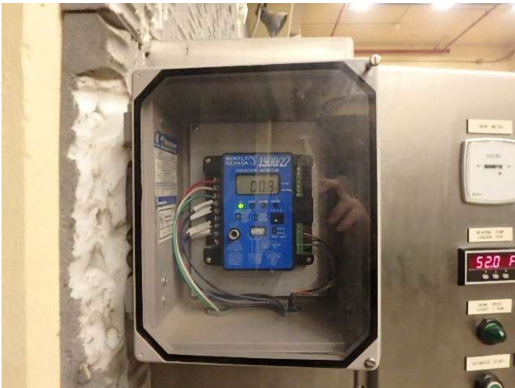
Centrifuge #2 Vibration Monitor
