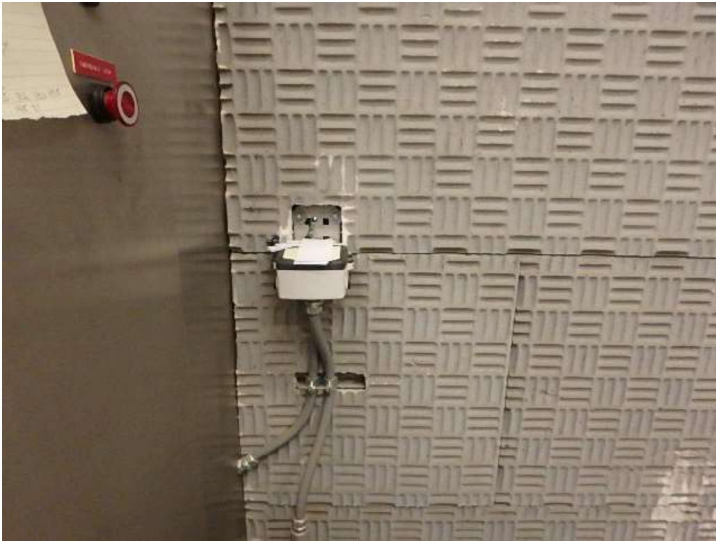
Centrifuge #2 Flowmeter Box Tie In
