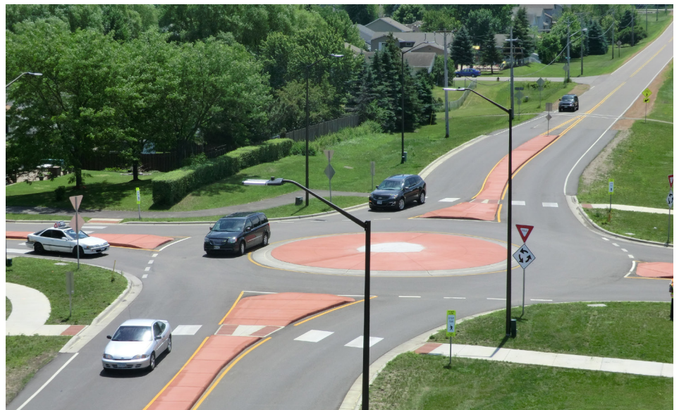
Example of a single-lane roundabout. Source: FHWA
