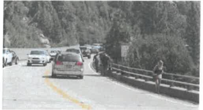
Pedestrians hug the viaduct's guardrail and walk in a 12- to 18-inch shoulder as they walk from their car to their destination.
