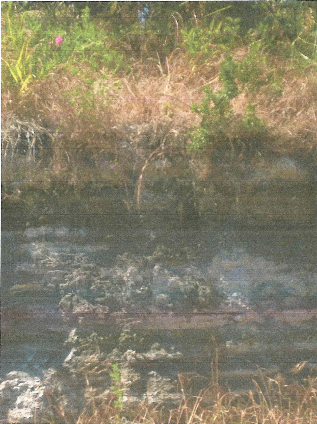
Facing South from the Lindeman property line looking at the bank on the Waste Connections property with just a small view of the layers of White Lime slag and pollutant on Waste Connections property that is at least 15 ft. above and extends UPHILL for several 100 yards under the Waste Connections MRF, old slag and slurry pits and holding ponds and beyond! 05/31/2016
