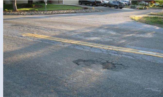
Before Chip Seal & Slurry Seal
