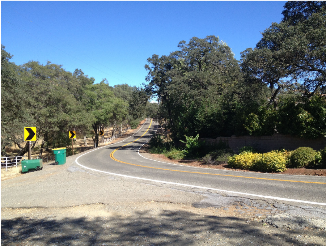
Figure 3.2-2(c): View from Just West of Existing Bass Lake Road Facing East Toward Proposed Intersection with Silver Springs Parkway
