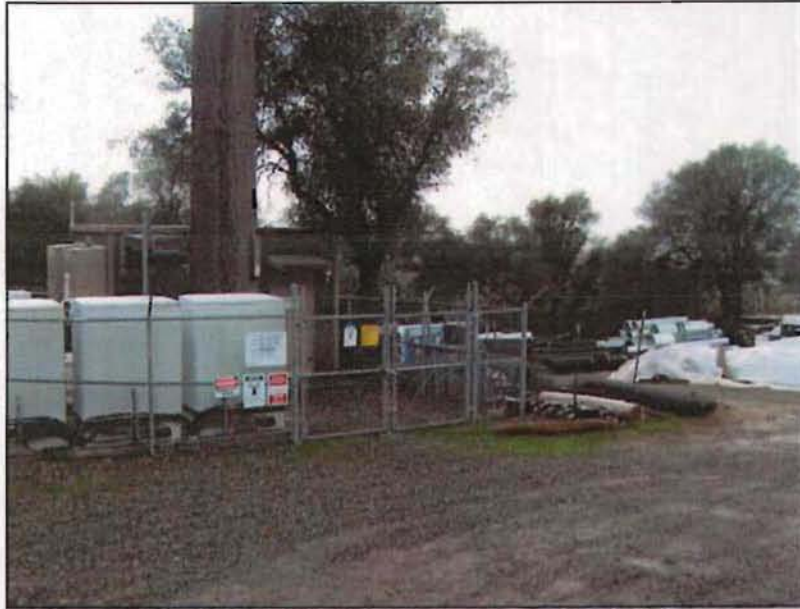
View of new utility site and tree #105 from northeast.
