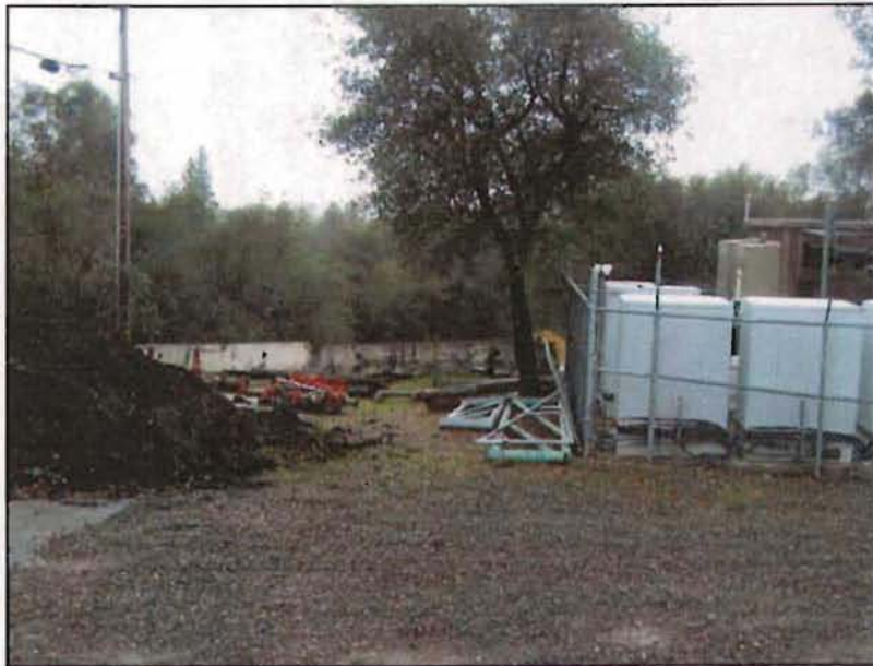
View of new utility site and tree #105 from east.
