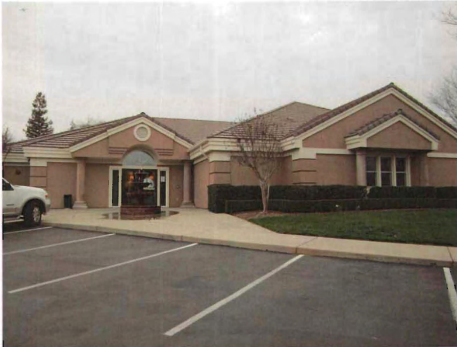
Existing Structure at Location of Addition
