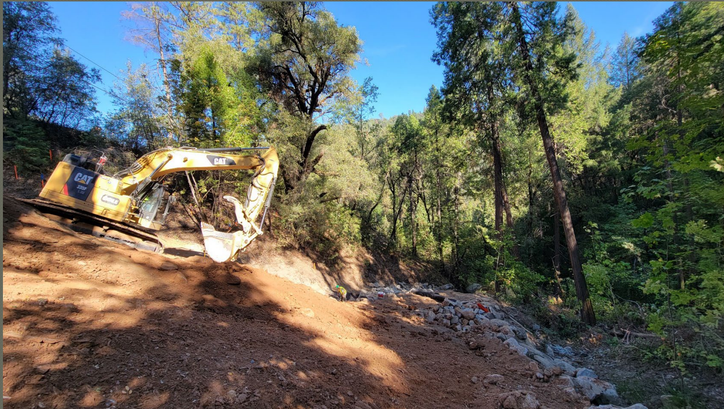
Drainage System #3 Rock Lined Ditch at South Approach
