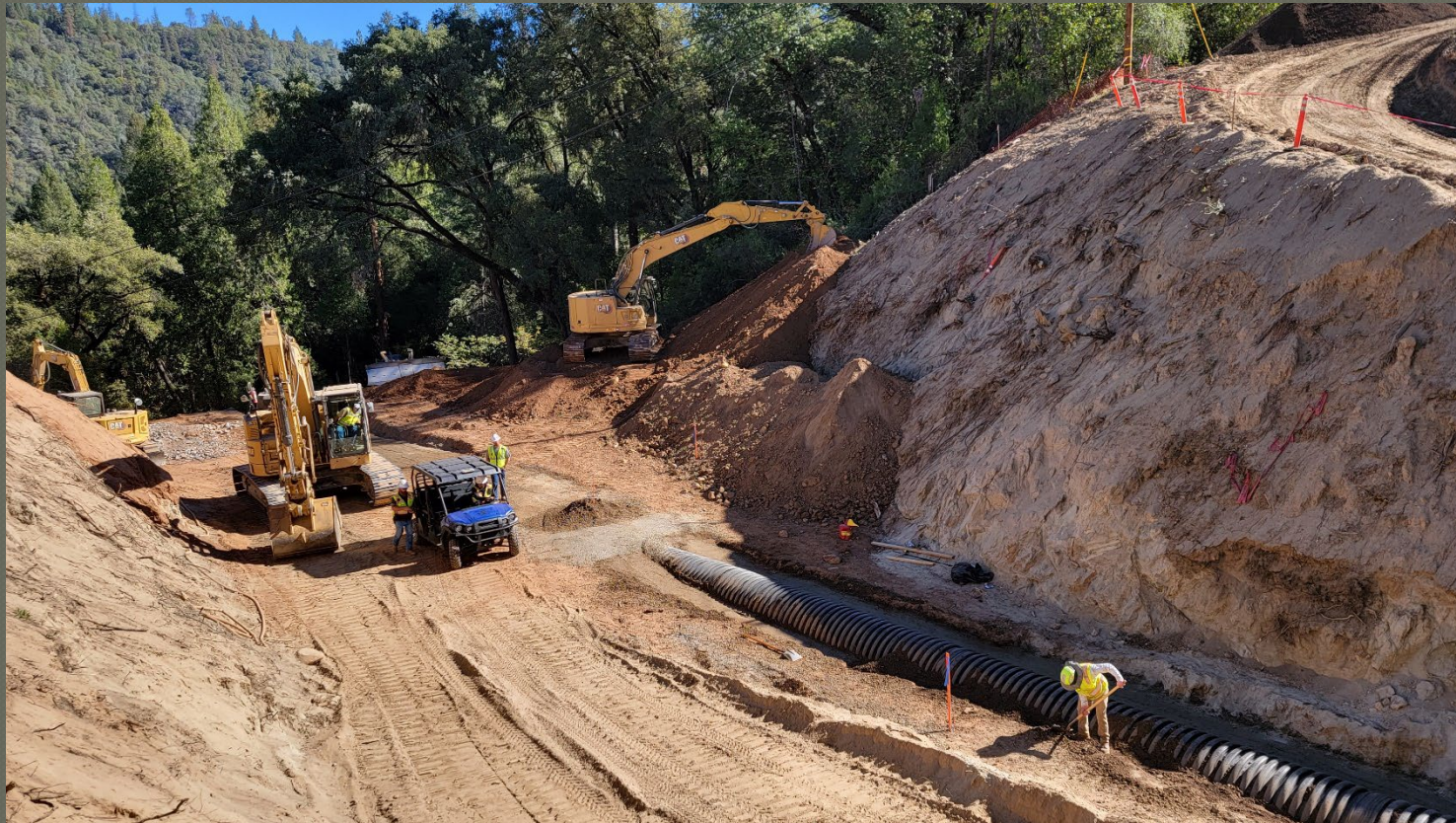
Drainage System #3 48" Pipe at South Approach
