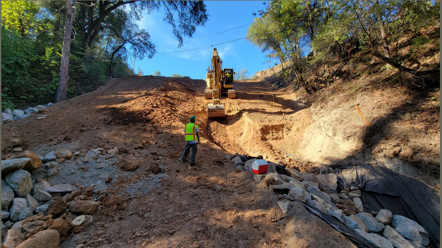
Drainage System #3 Rock Lined Ditch at South Approach
