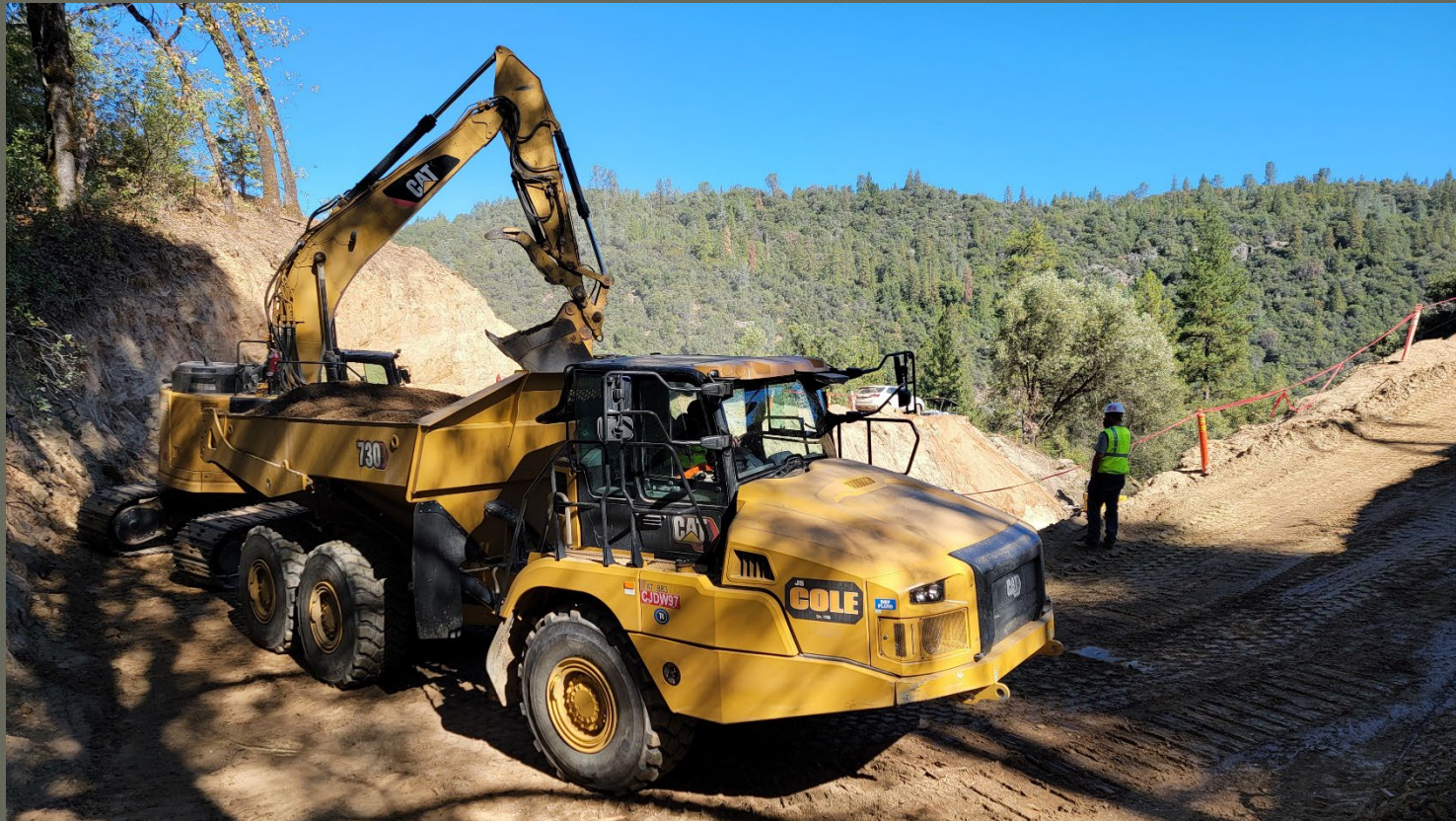
Construction Access Road at South Approach
