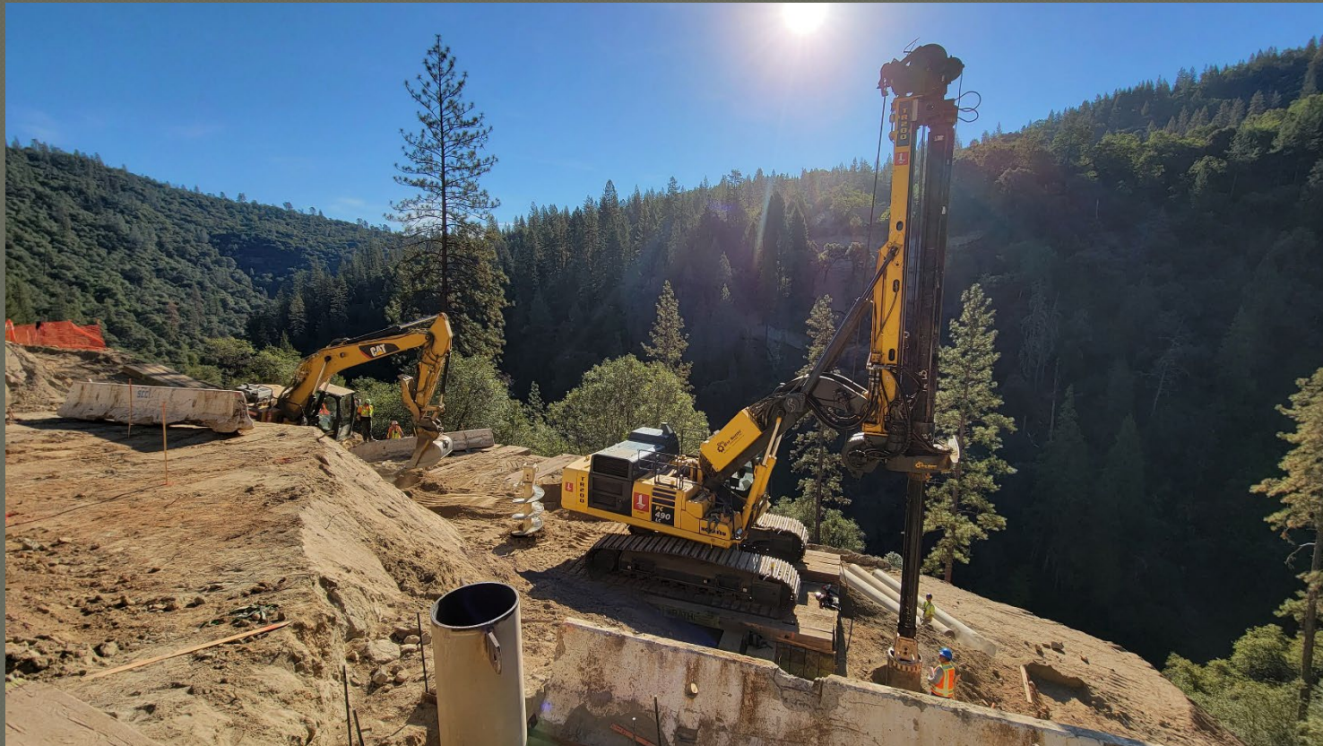
Drilling Foundations for Trestle at North Side
