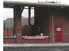
Household hazardous waste collection area
