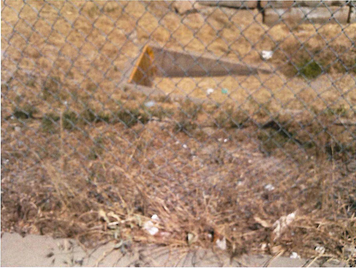
Outlet Drains from pond #2 concrete lined ditch
