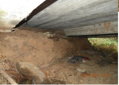
Bridge girder foundations show signs of undermining
