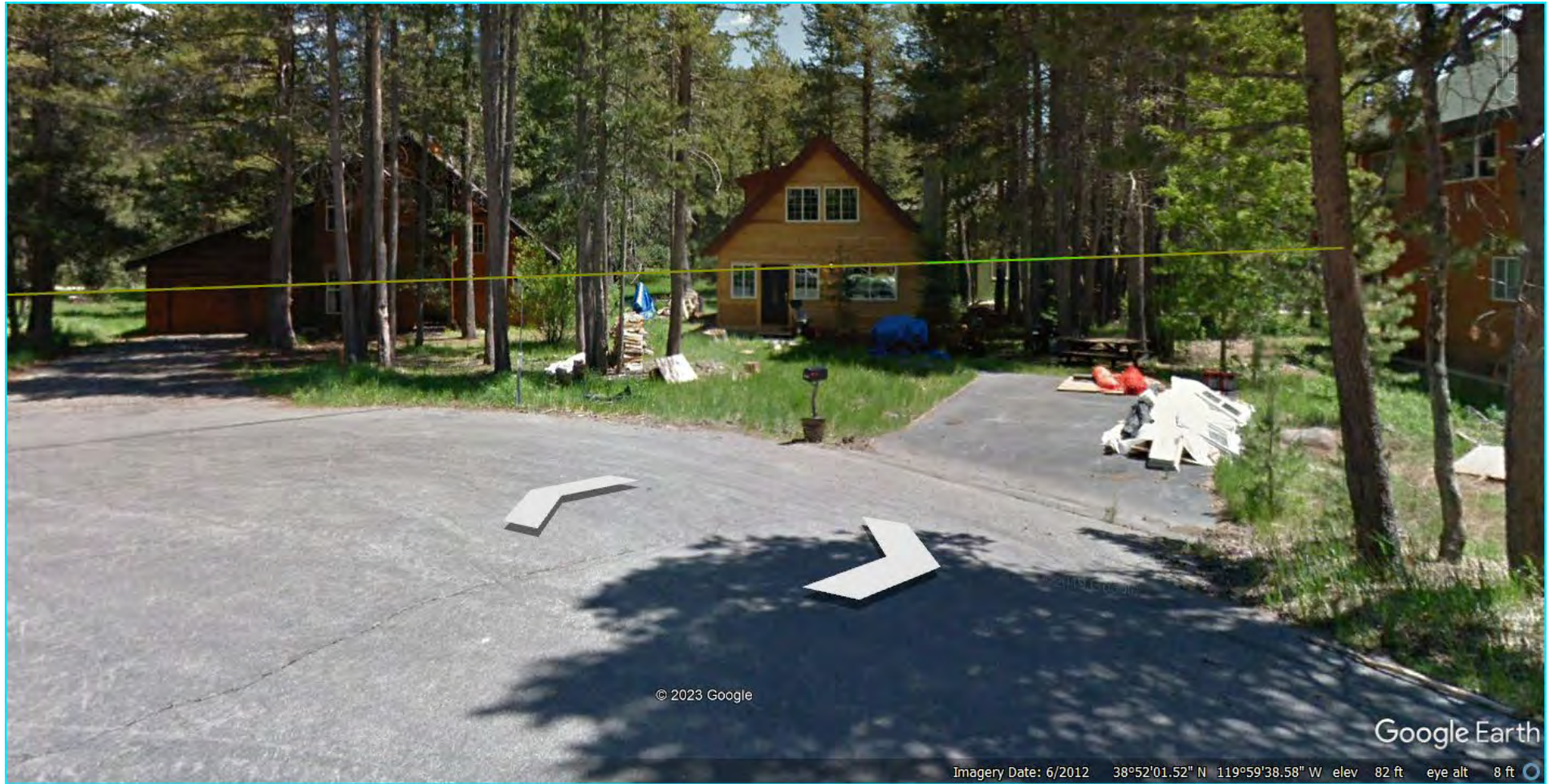
Exhibit F - Existing Conditions
