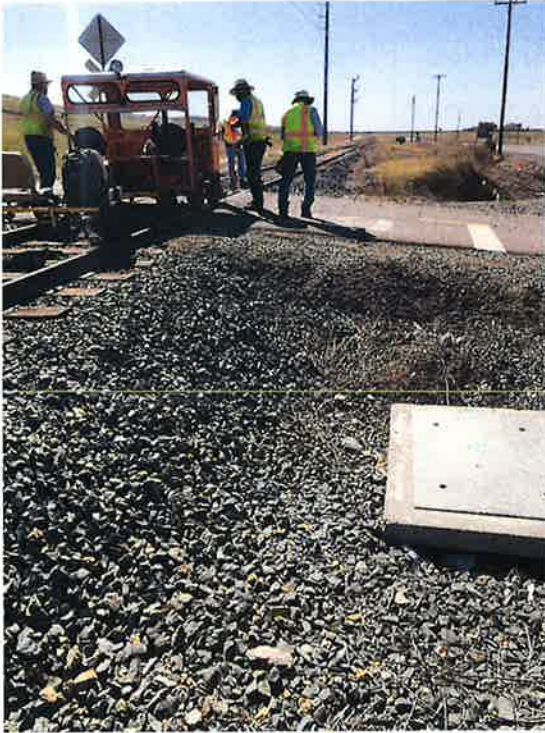
Drain installed next to tracks creates an excessive slope in walkway.
