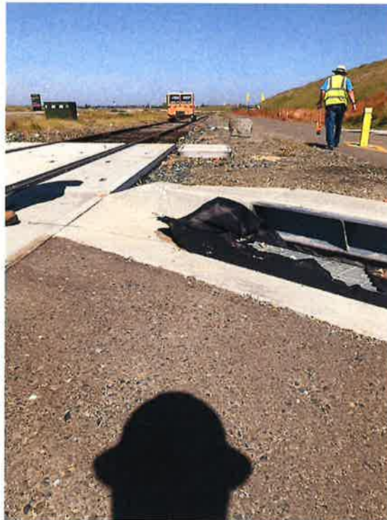
New crossings installed create multiple tripping hazards in the walkway (raised utility boxes, curb raised above sidewalks and roadway, crossing pads not filled in with ballast, and large rocks)
