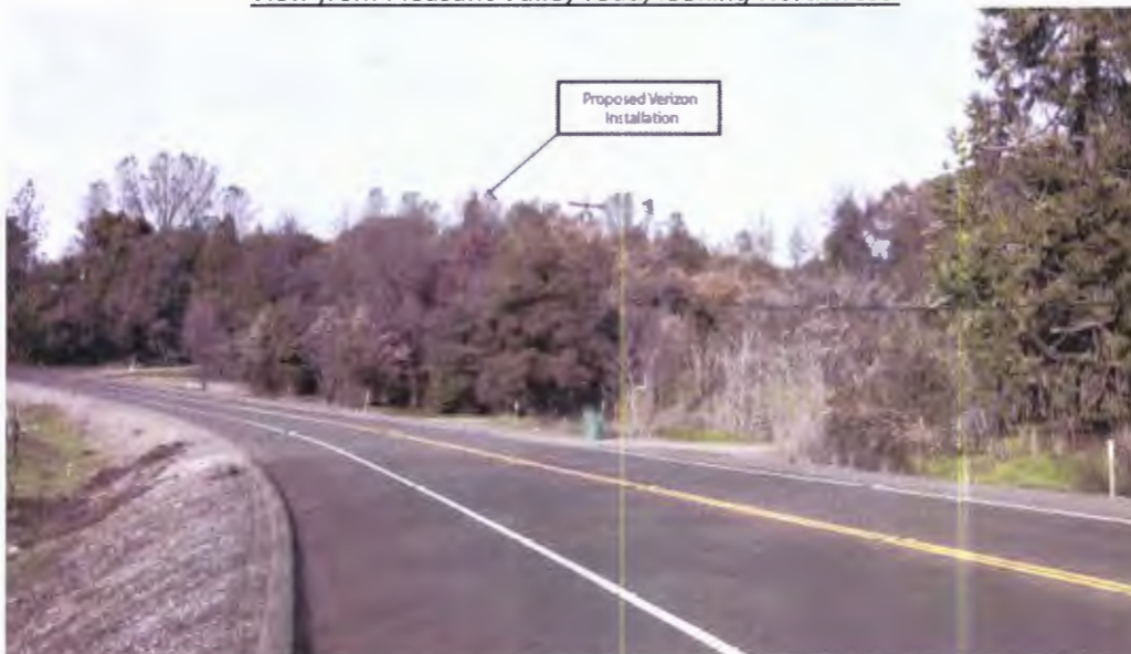
View from Pleasant Valley road, looking Northwest:
