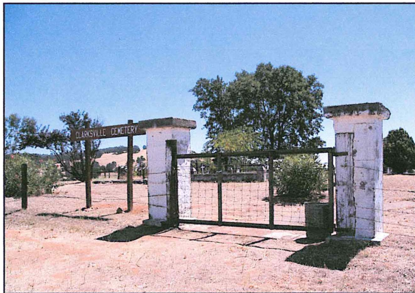
Existing gate and barbed wire fencing.
