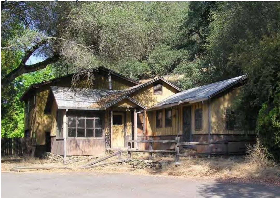
Figure 6 Residential Building, looking West
