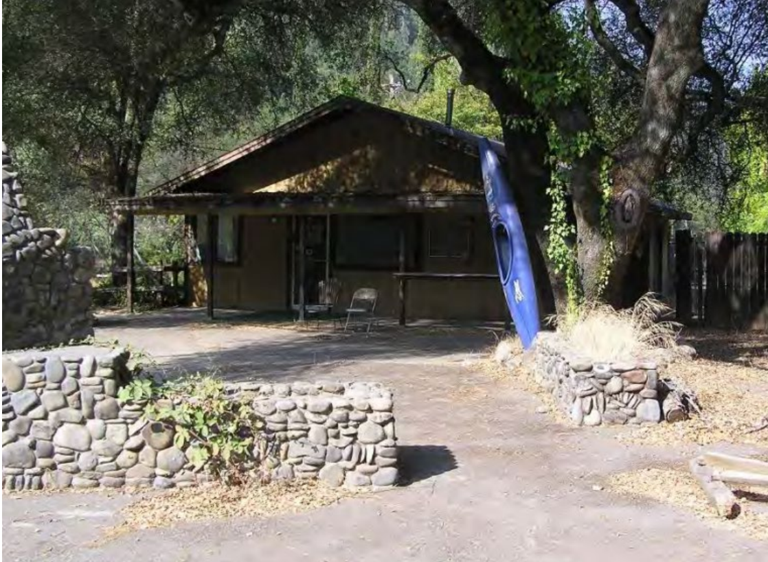
Figure 5 Store Building, looking West
