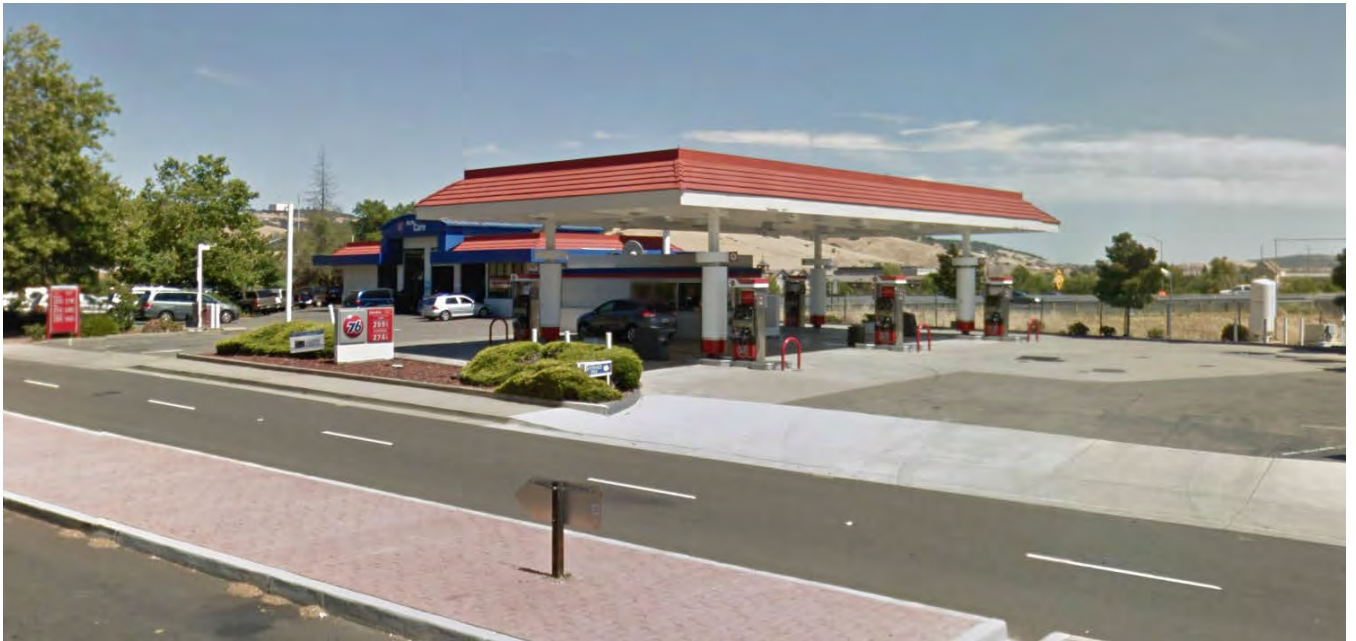
Existing canopy (view from Saratoga Way)
