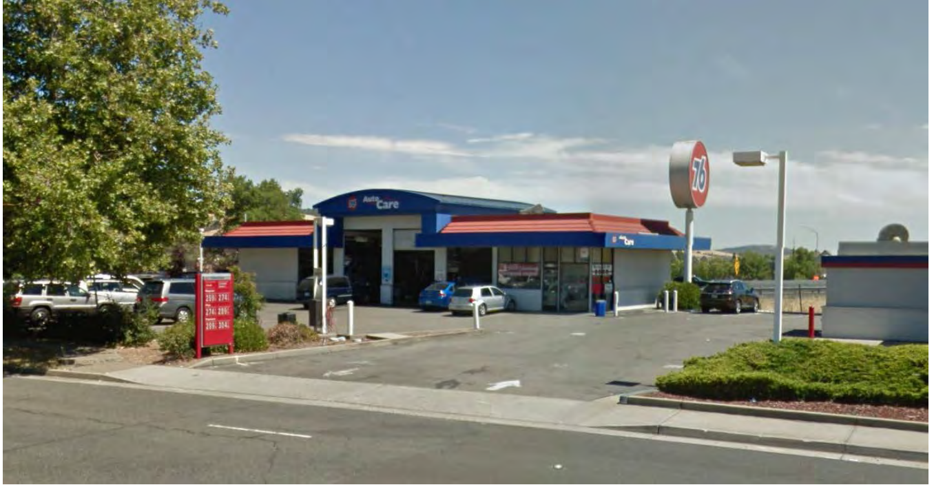
Existing Auto service building (view from Saratoga Way) Convenience store addition to match existing building
