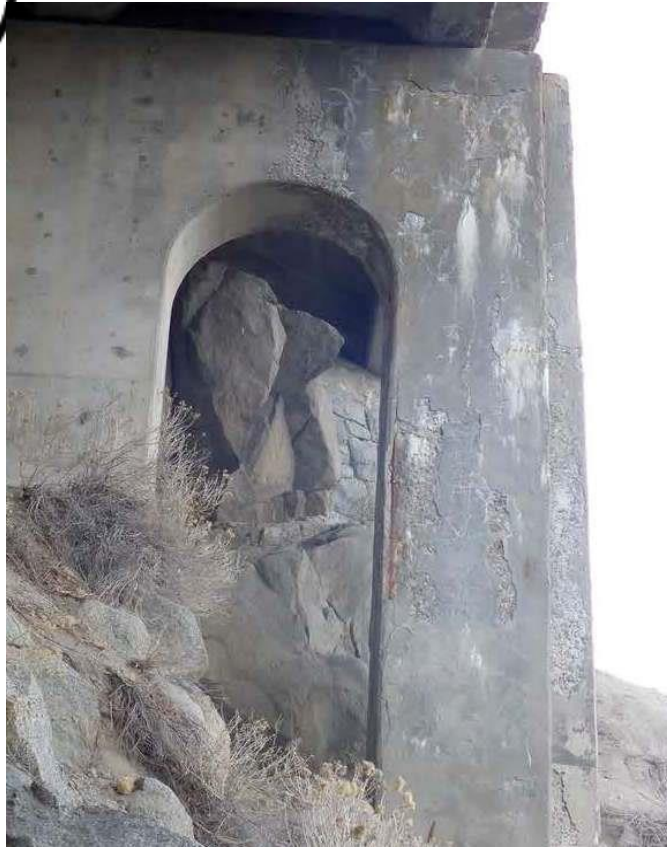
Concrete spalling and exposed rusted reinforcing steel in piers
