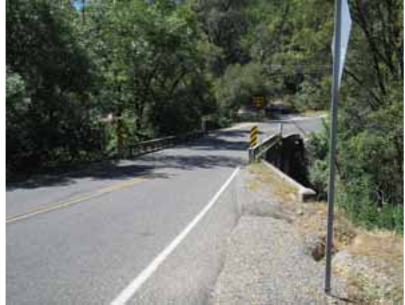
Photo 2. View looking south along Green Valley Road Bridge. 6 June 2008
