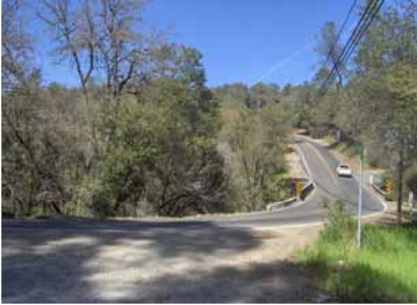
Photo 1. View looking north along Green Valley Road Bridge from Lode Road. 27 March 2008
