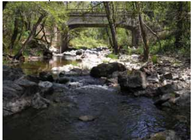
Photo 6. View looking east downstream of the Green Valley Road Bridge. 25 April 2008
