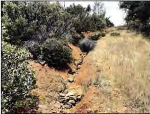
Constructed drainage running north/south through the eastern portion of the property.
