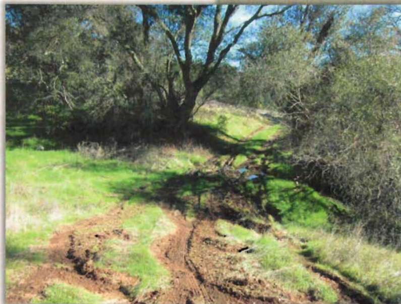
Proposed driveway location at first culvert placement. 2 oak trees (right side of photo) will be removed.
