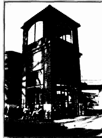
The Village Center at 19th and S Streets in Sacramento successfully illustrates the concept of base-middle-cap. The base of the structure is accented with a stone material. The mid section is brick, and the top is stucco.
