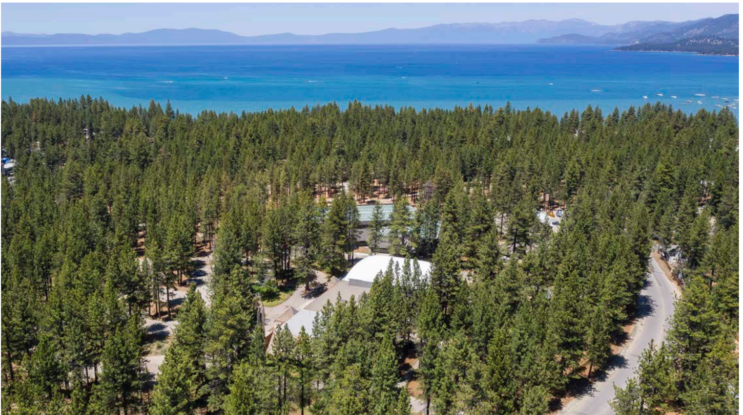
Rufus Allen Boulevard with the existing Recreation Center in the foreground.
