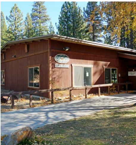
Existing buildings on site.
