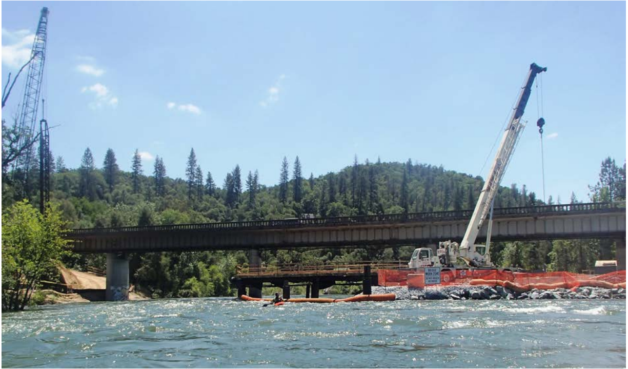
Photo 6. Hwy 49 Replacement Bridge construction
