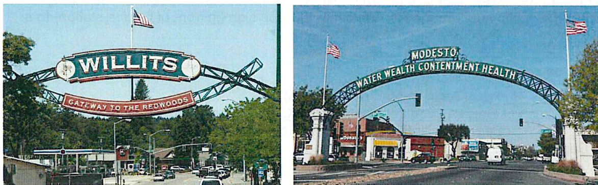
Figure 28. Gateway arches in Willits and Modesto, CA.
