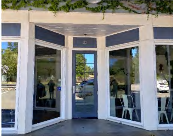
Figure 29 Commercial Windows and Doors
