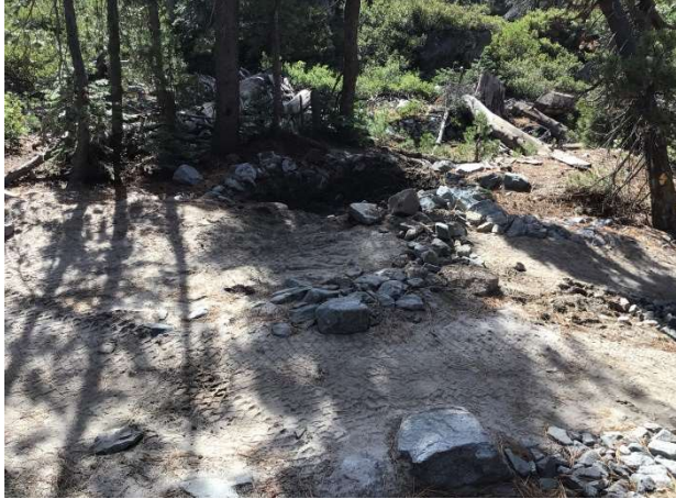
Photo of BMP work in progress
