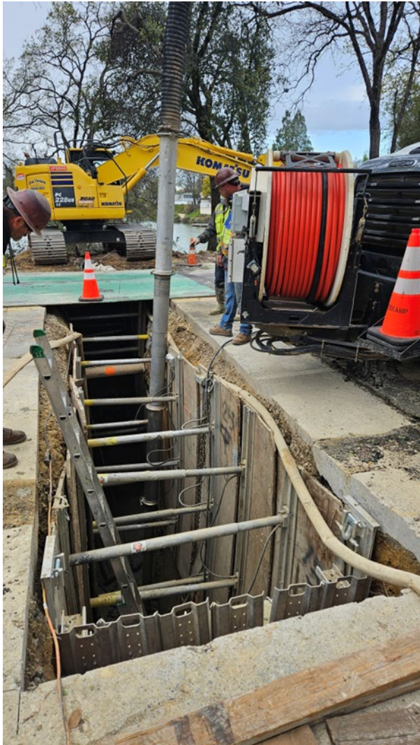
15' deep culvert excavation under Patterson Drive
