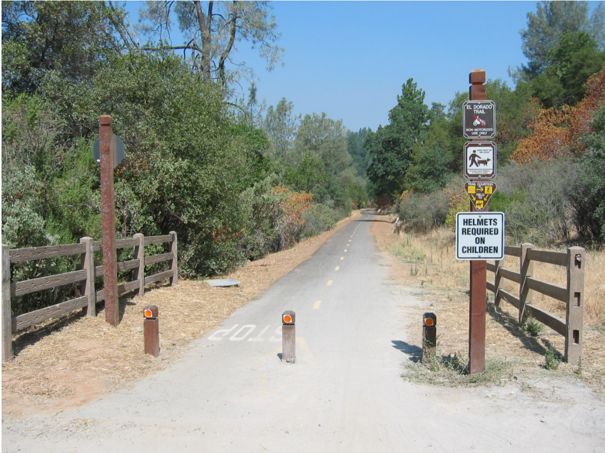
End of Improved Portion of El Dorado Trail at Los Trampas Drive
