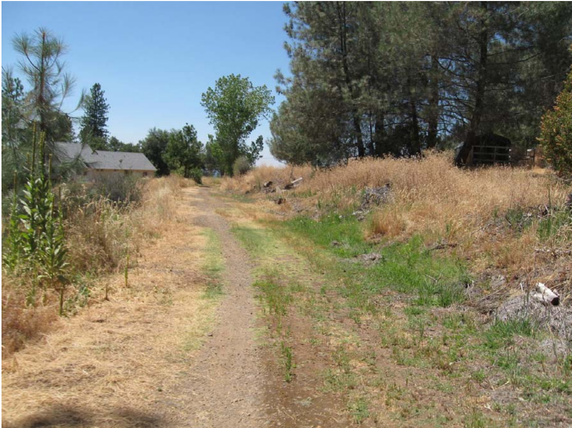
Typical cross-section of Project site. Trail surface varies from dirt, to mud, to grassy vegetation, to gravel, to a thick layer of previously installed railroad ballast.
