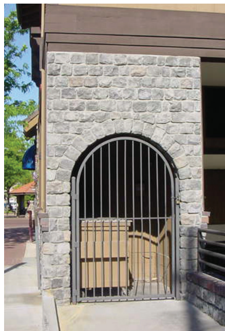
Utilities should be screened with landscaping
