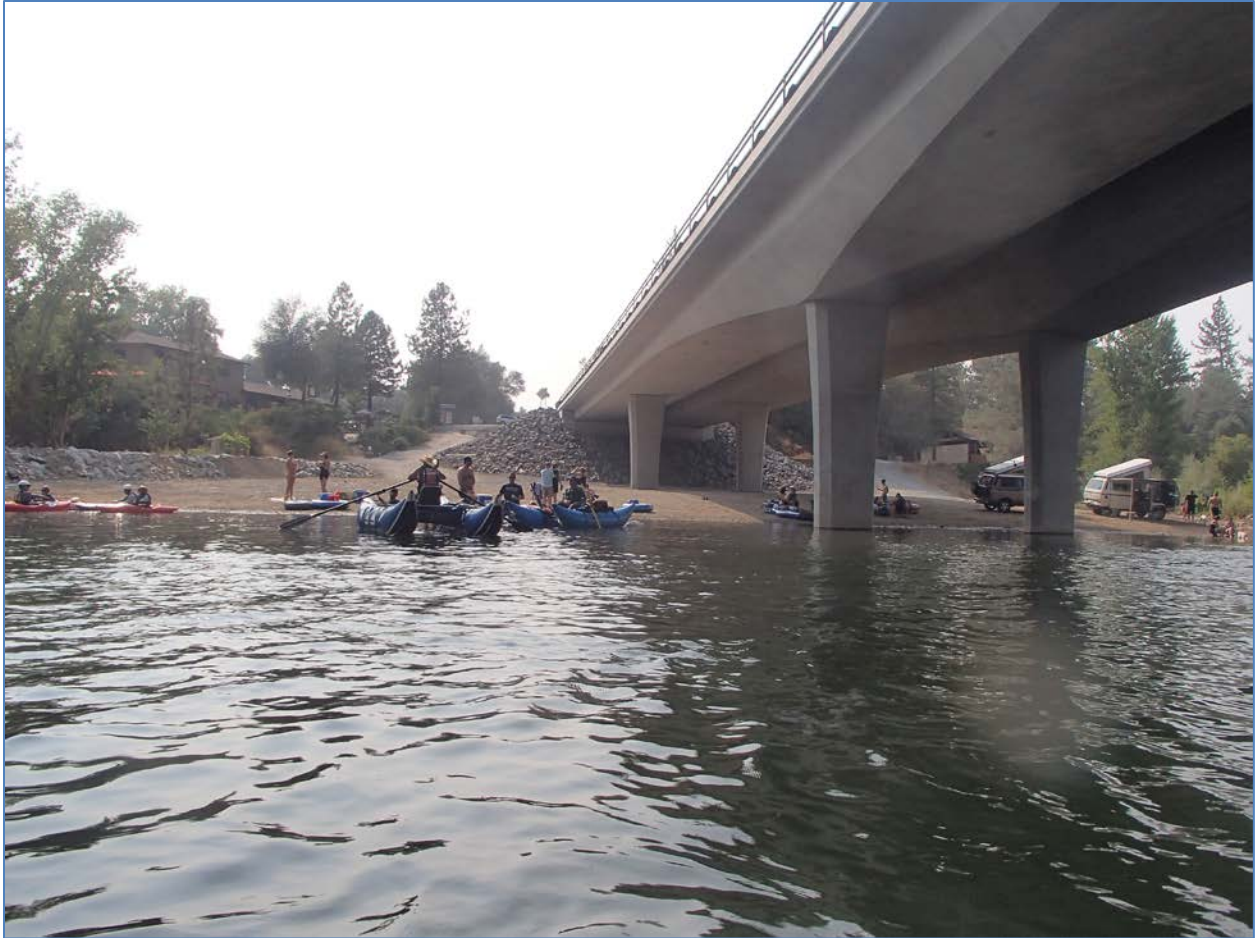
Photo 5. People enjoying the river by the newly completed Hwy 49 Replacement Bridge
