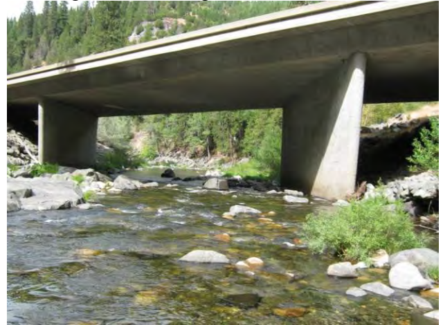
Looking N under bridge
