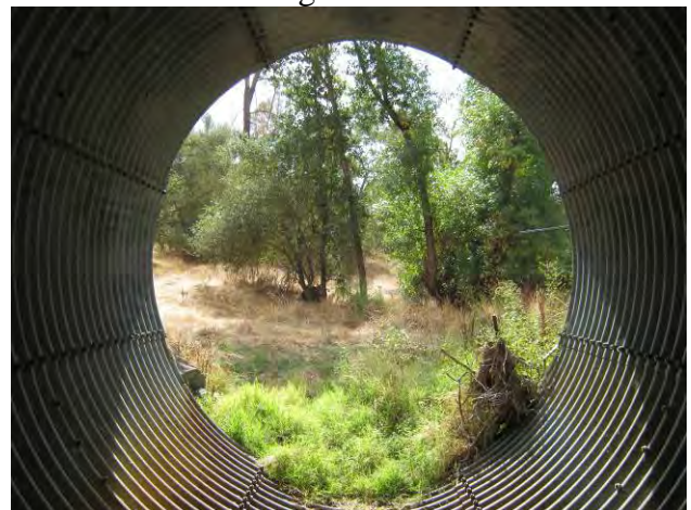
Inside culvert looking South
