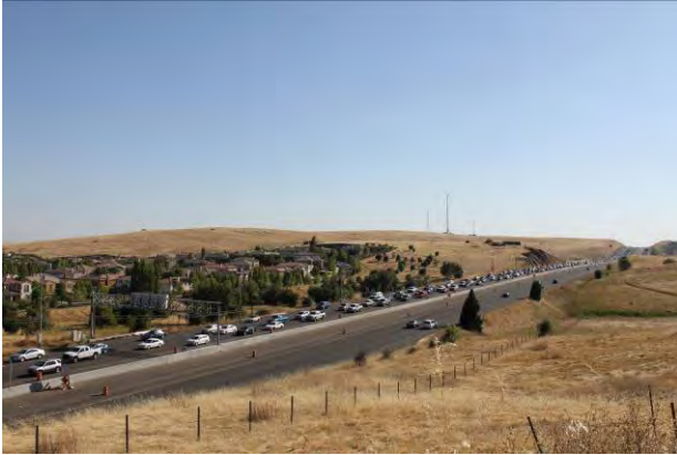
Westward landscape view toward culvert
