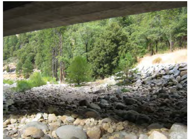
View North under bridge and adjacent vegetation
