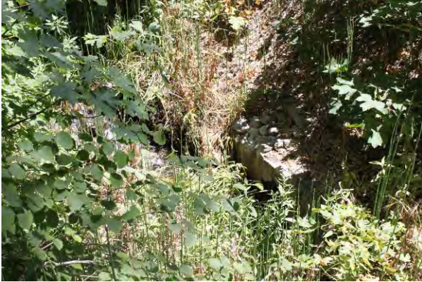
Close-up view of opening on North side
