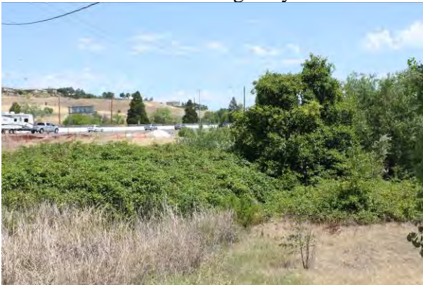
Eastward medium view highway culvert
