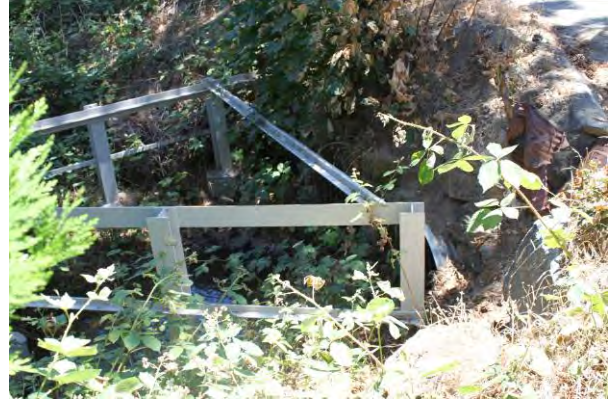
Close-up view North side
