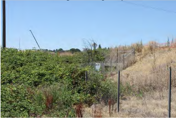
Westward close-up view highway culvert
