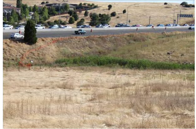
Westward closer view toward culvert
