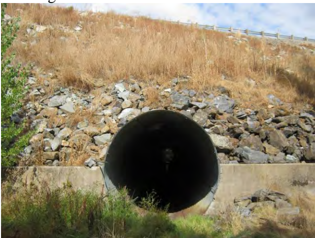
Looking North toward culvert
