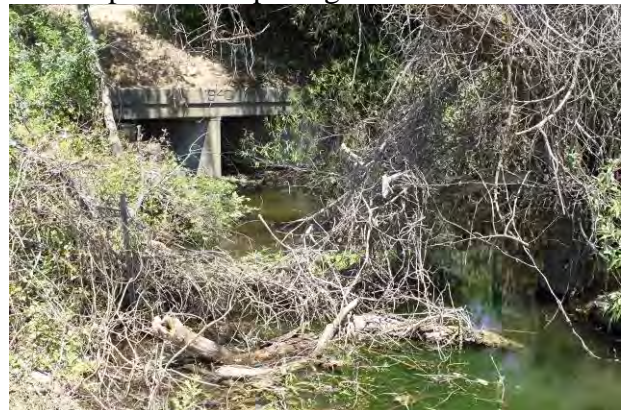
Close-up view of opening
