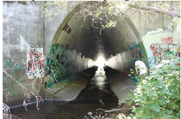
Close-up view of culvert opening
