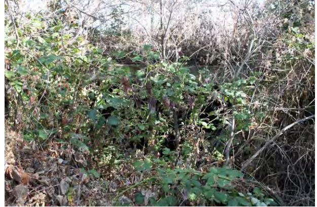
Close-up view of opening
