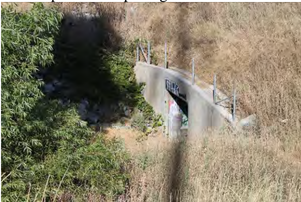
Close-up view of opening
