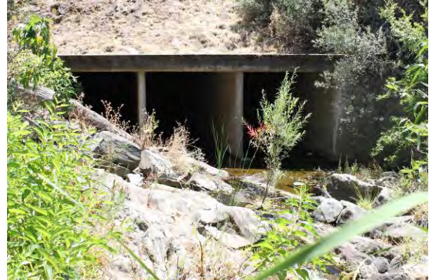
Close-up view of opening
