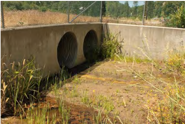
North side of culvert
