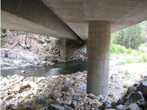
View under bridge looking West
