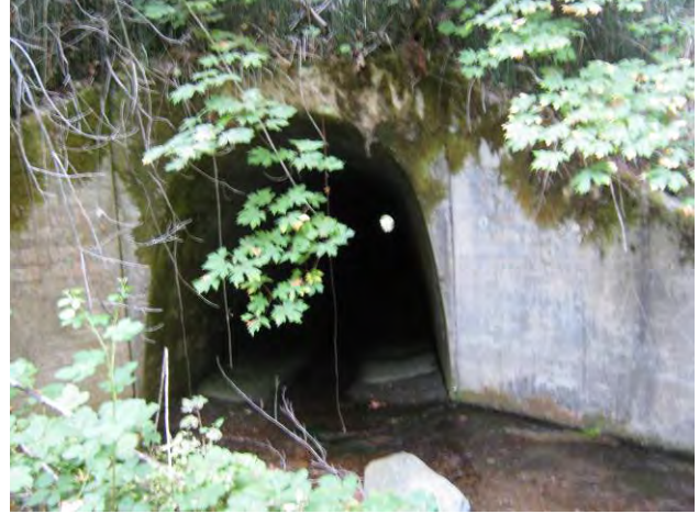
Looking into Southern entrance (Northern end visible as point of light)
