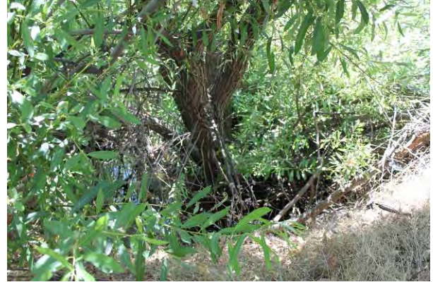
Close-up view from above of opening
