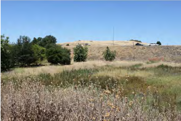
Westward medium view toward culvert
