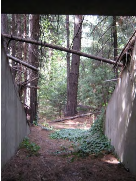
North end view from tunnel
