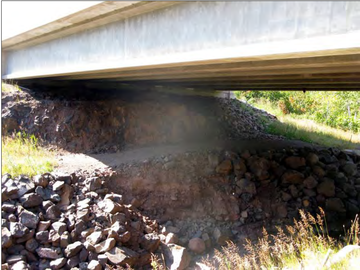
Figure 13. Level Walkway Added Under Existing Highway Bridge in Northern Minnesota to Facilitate Lynx Crossing
