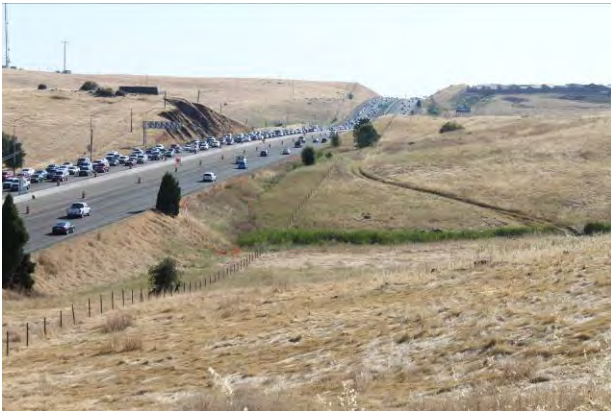
Westward medium view toward culvert
