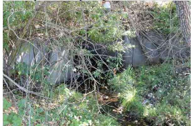
Close-up view of opening
