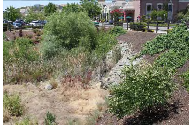
Westward close-up view second culvert
