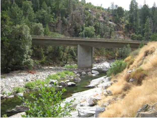
View under bridge from North
