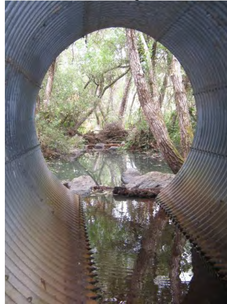
Inside culvert looking North
