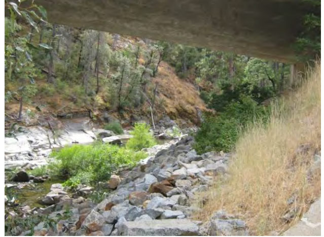
Rip-rap on West bank of under-crossing
