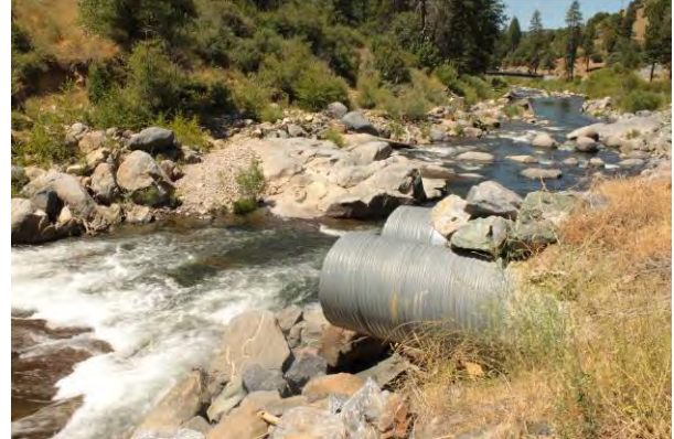
South side of culvert
