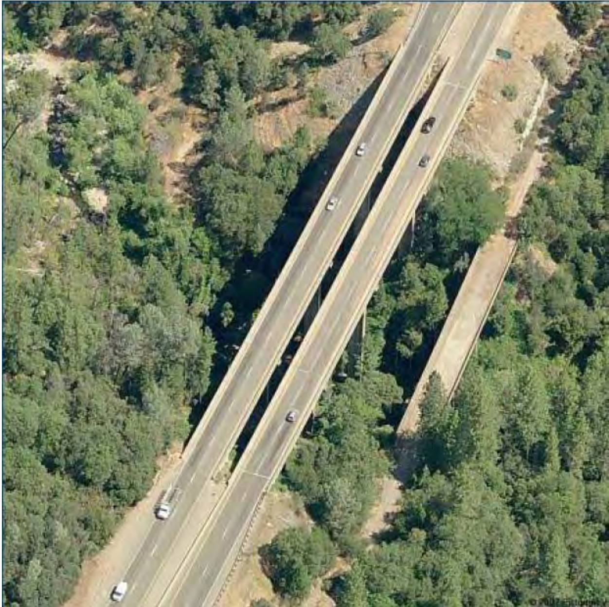
Figure 9. Weber Creek Under-Crossing
