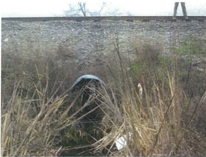
Feature 9: This feature is a corrugated steel culvert surrounded by rock. Facing north
