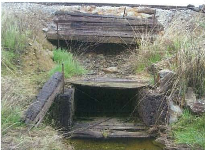
Feature 11: This feature is a wooden culvert constructed of railroad ties with erosion control of railroad ties above. Facing South. Frame 3314.
