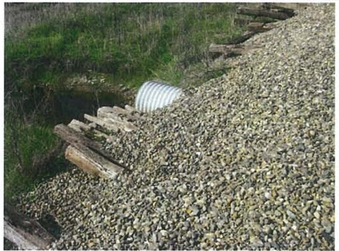
Feature 74: This feature is a corrugated metal culvert with railroad ties above for erosion control. Facing W. Frame 3474.
