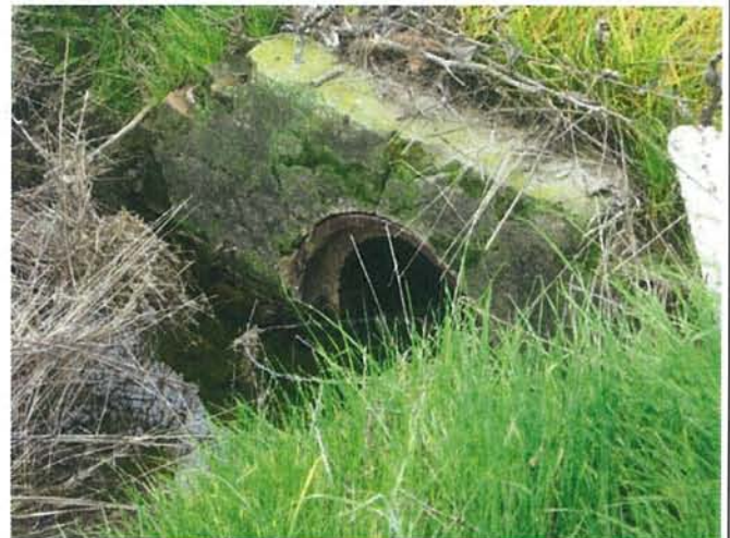
Feature 24: This feature is a culvert of brick encased in mortar surrounding a brown glazed ceramic culvert with "...LINCOLN, CA" stamped on the mouth of the ceramic. Facing S. Frame 3332.
