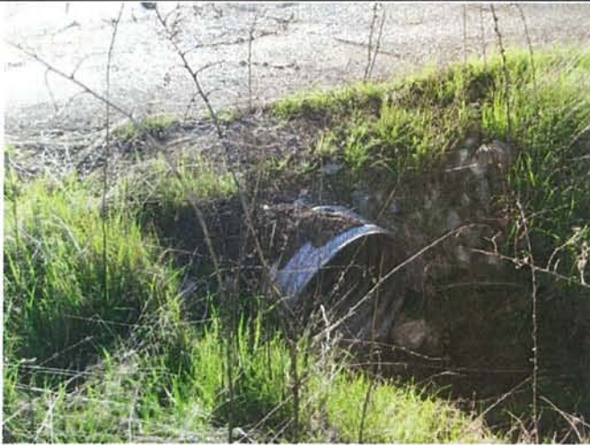
Feature 5: This feature is a corrugated metal culvert. Road repaved above. Facing W. Frame 3350.
