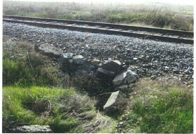
Feature 6: This feature is rock and steel pipe culvert. Facing W. Frame 3305.
