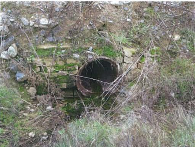
Feature 15: This feature is a brown glazed ceramic culvert surrounded by brick. Facing WSW. Frame 3320.
