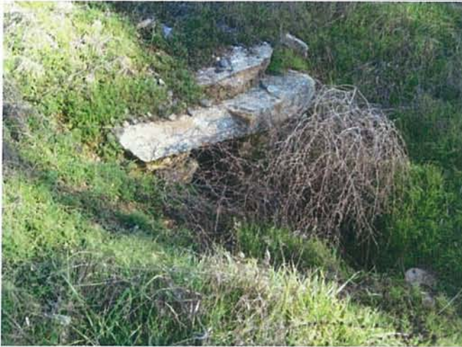
Feature 53: This feature is a small square stacked greenstone culvert. Facing SE. Frame 3422.
