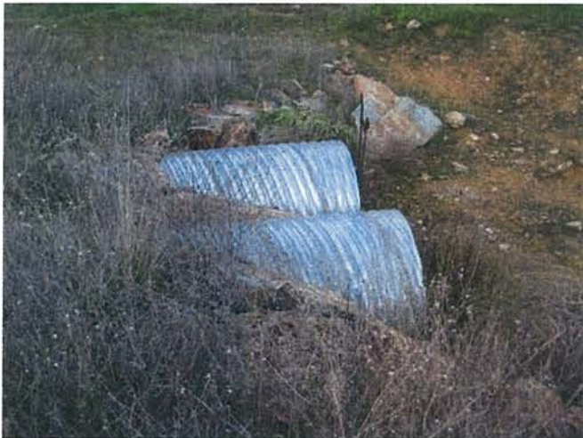
Feature 63: This feature is a double corrugated metal culvert. Facing NE. Frame 3443.
