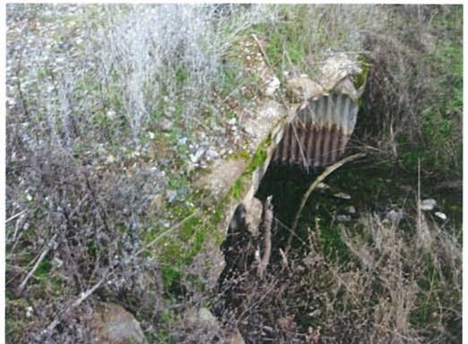
Feature 64: This feature is a double corrugated metal culvert with concrete sandbags. Facing N. Frame 3444.
