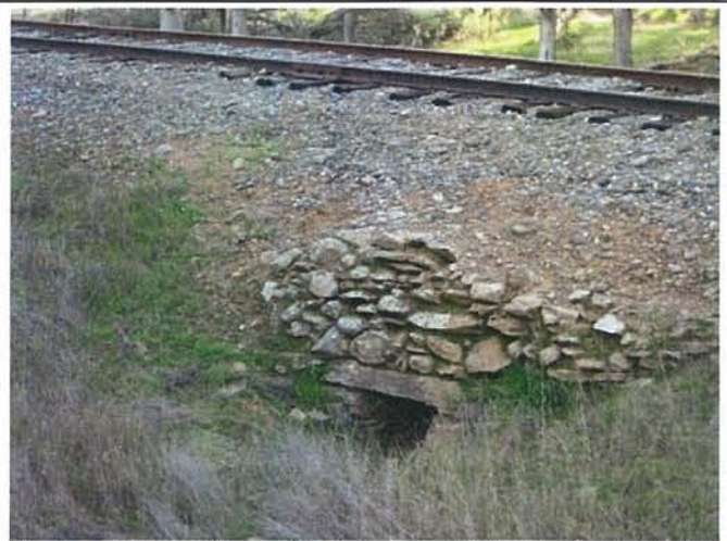
Feature 58: This feature is a greenstone culvert with multiple courses of greenstone stacked on top. Facing N. Frame 3433.
