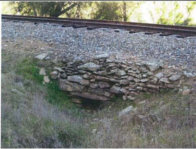
Feature 57: This feature is a stacked greenstone culvert with multiple courses of greenstone stacked on top. Facing N. Frame 3432.
