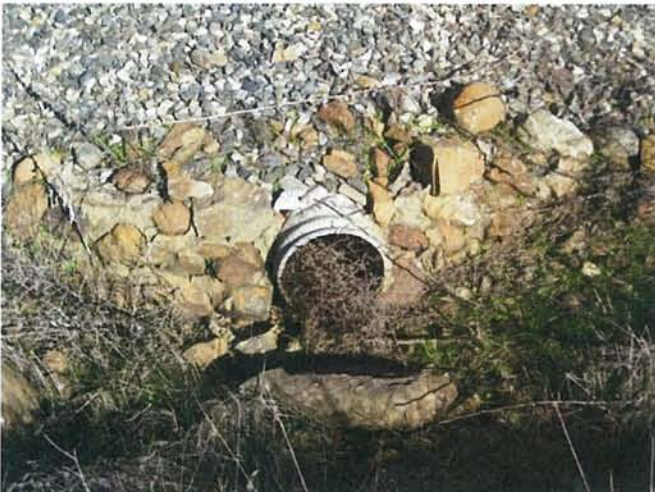
Feature 87: This feature is fieldstone and loose mortar around a corrugated metal culvert. Facing ENE. Frame 3495.
