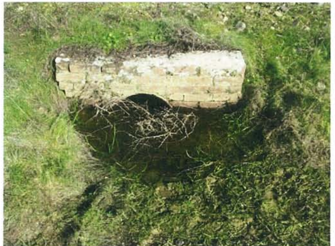
Feature 84: This feature is a clay culvert surrounded by brick and mortar. Facing ENE. Frame 3491.
