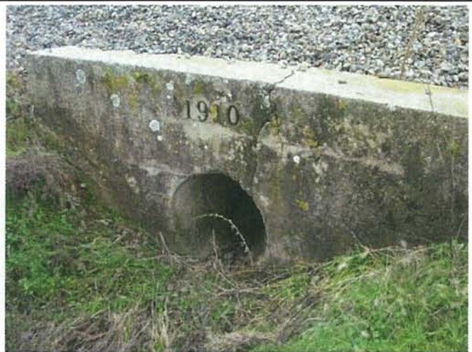
Feature 26: This feature is a poured concrete culvert with a date of "1910" stamped onto the face of the concrete. Facing S. Frame 3338.
