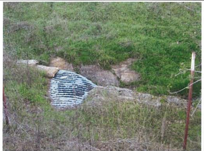
Feature 62: This feature is a very large corrugated metal culvert with cement sandbag support. Facing NE. Frame 3441.
