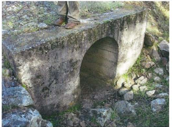
Feature 34: This feature is a poured concrete arched culvert. Facing N. Frame 3389.
