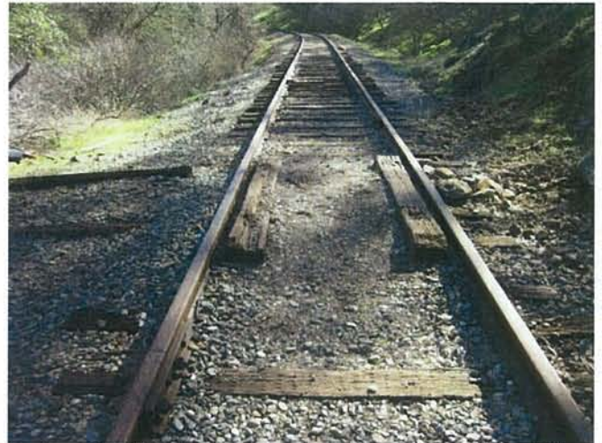
Feature 38: This feature is a wooden de-railer track at which hand cars come off the track. It is comprised of one set of parallel embedded railroad ties in between the tracks themselves that are nine feet long, and two parallel embedded railroad ties 5 feet apart coming jutting out from the track for 14 feet. Facing ESE. Frame 3396.
