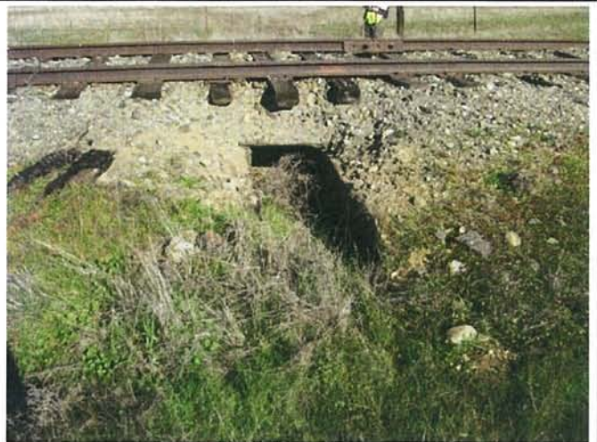
Feature 86: This feature is a burnt out wooden culvert. Facing ENE. Frame 3494.
