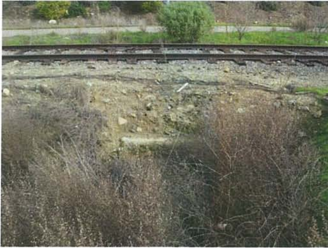
Feature 1: This feature is a concrete capped corrugated metal culvert. Facing E. Frame 3297.
