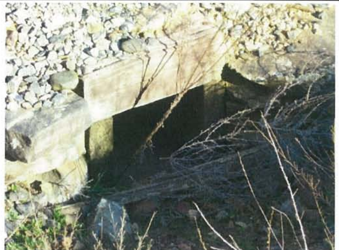
Feature 54: This feature is a very small wooden culvert. Facing E. Frame 3423.
