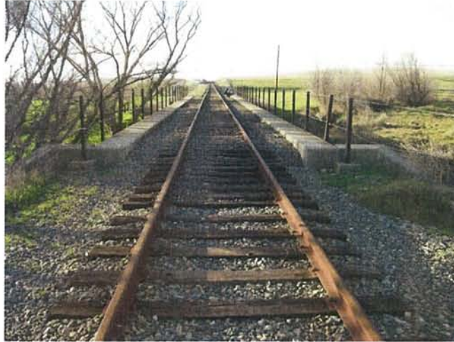
Feature 91: This feature is a concrete bridge 134 feet long and 17 feet wide with a 2.5 foot wide concrete foot path on either side, and a railing made of 3.5 foot tall metal posts strung through with thick wire. It has 4 concrete piers and is supported by concrete abutments. Photo facing NW. Frame 3364.
