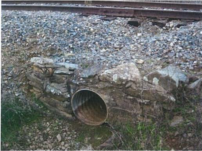
Feature 65: This feature is a corrugated metal culvert encased in mortared courses of angular rocks. Facing NE. Frame 3445.
