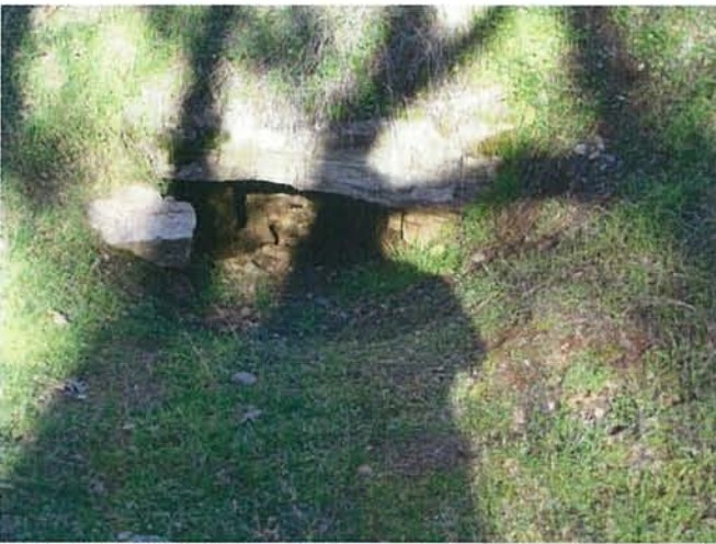
Feature 47: This feature is a large, stacked greenstone culvert. Facing NE. Frame 3416.
