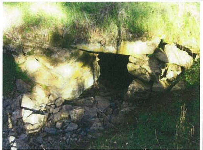
Feature 46: This feature is a large stacked greenstone culvert. Facing NE. Frame 3415.
