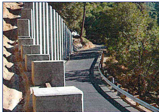
Soldier Pile Wall Constructed in 2007
