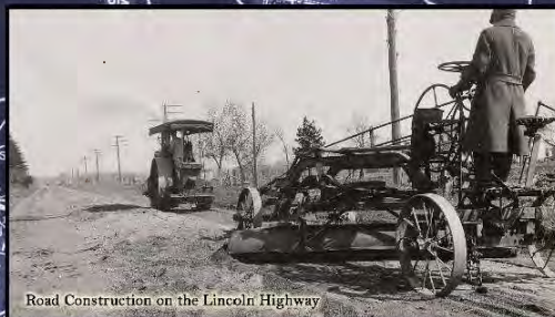
Road Construction on the Lincoln Highway
