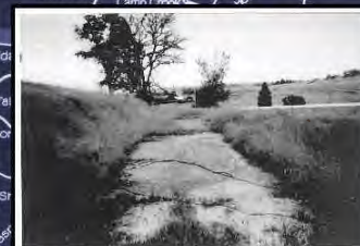
Barb wire blocks the old Lincoln Highway off Bass Lake Road south of US 50. Kathy Franzwa
