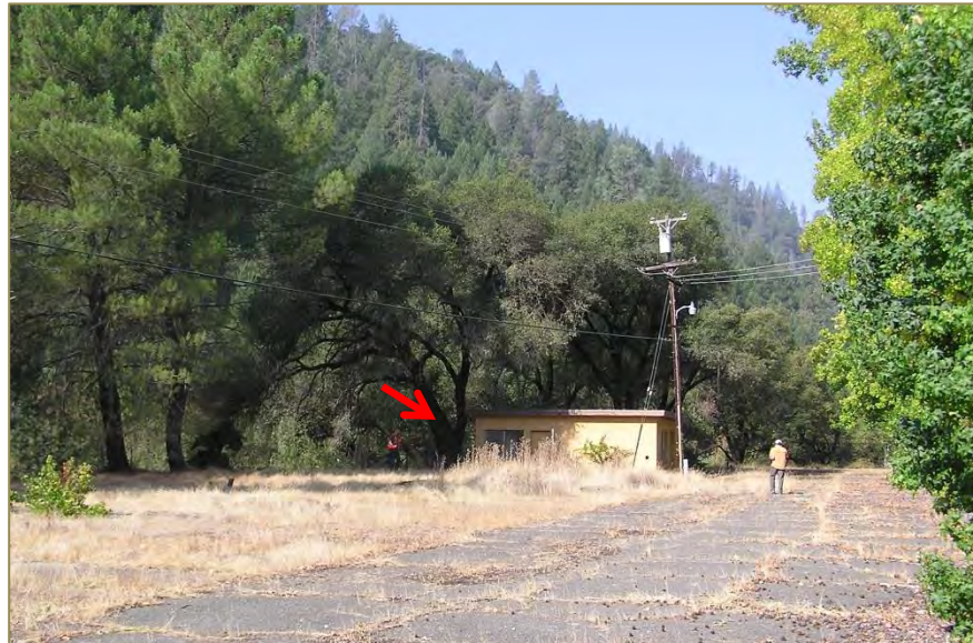
Exhibit IV-1 Existing Restroom Build at Former Mobile Home Area
