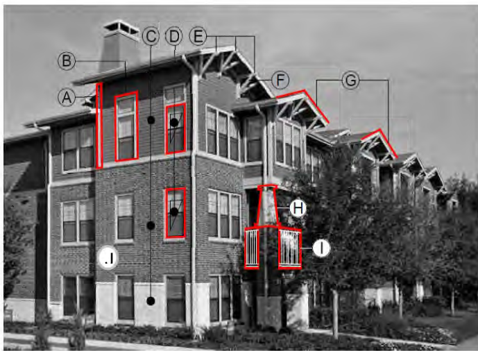
Figure 2. Typical Design Features of the Railroad Craftsman Style
