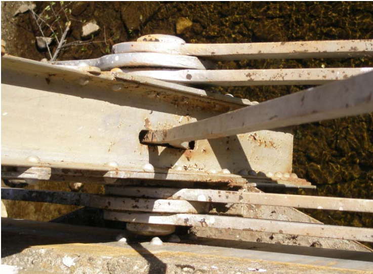
Figure 2 - Fracture critical diagonal eye-bar truss
