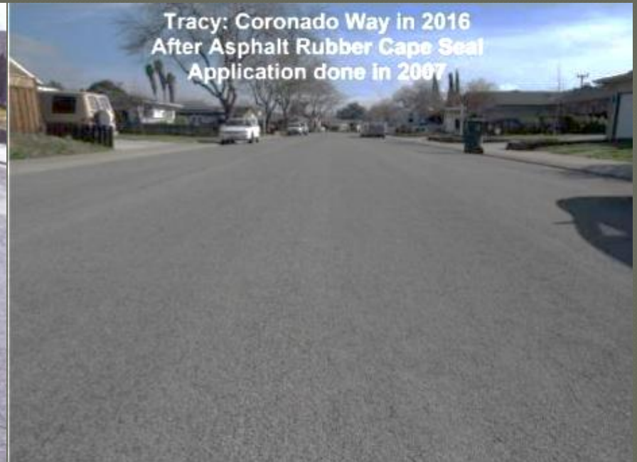
2016 – After Rubber Cape Seal Application completed in 2007
