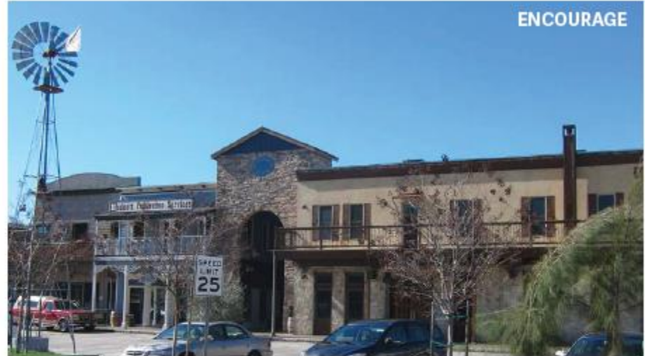
This new mixed-use building uses facade materials similar to those used in historic buildings. The different facade treatments help break up the long building.
