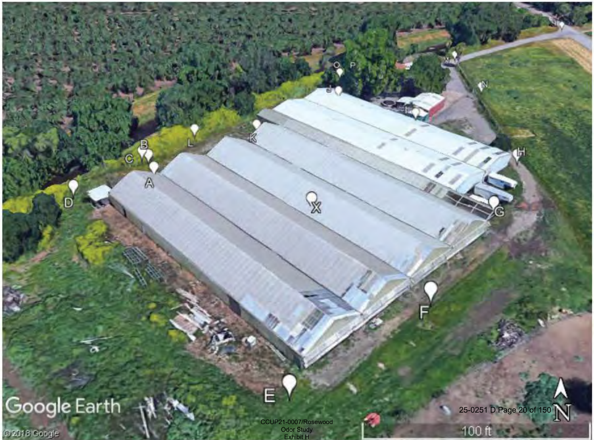
Figure No. 3 - Onsite Odor Inspection Locations (Google Earth Map)
