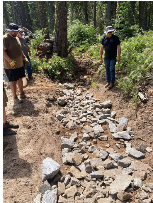
Rock outlet after clearing
