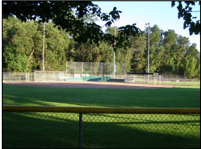
Existing lighted ballfield at HLP
